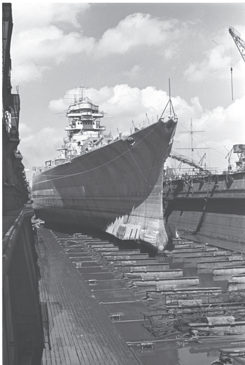
Blohm & Voss shipyard, Hamburg, late June – early July 1940. Bismarck is sitting in the floating dry dock No.V–VI. Not all the braking shields have been removed from the ship's bottom yet. Bismarck 's bow is already reconstructed to the curved 'Atlantic stem', and the main armour belt is in place as well. At the very bottom of the bow section there is a circular cover visible. Behind it is the Bugspiere , an extensible rod to which paravanes would be attached during operation. (Bundesarchiv, Bild 193-29-2-32)
