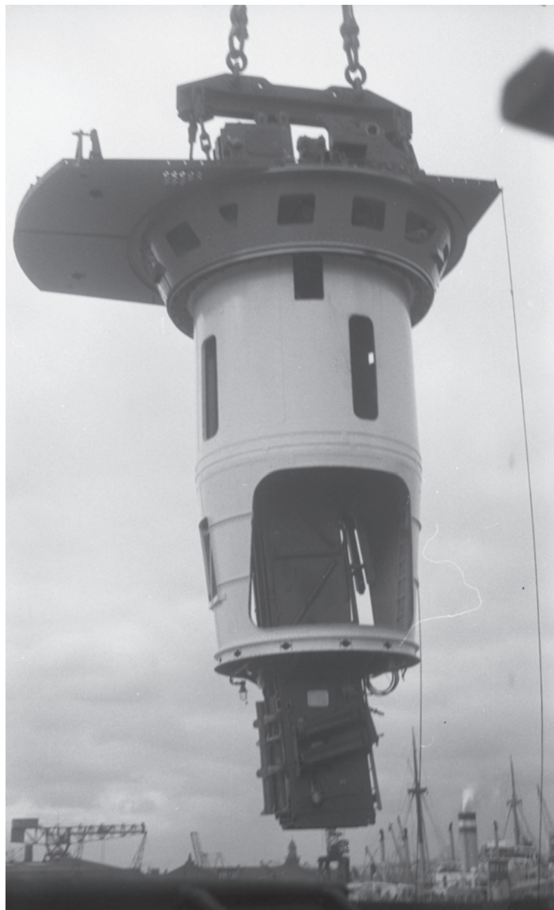
Blohm & Voss shipyard, Hamburg, 1939. A secondary turret is lowered by a crane to its position inside the barbettes. At the very bottom (ammunition handling level), the shell loading point and propellant cartridge loading point are visible. By the height of the turret, it can be determined that this is one of the fore turrets (either Stb I or Bb I). ( Bundesarchiv, Bild 193-34-1-05A )
