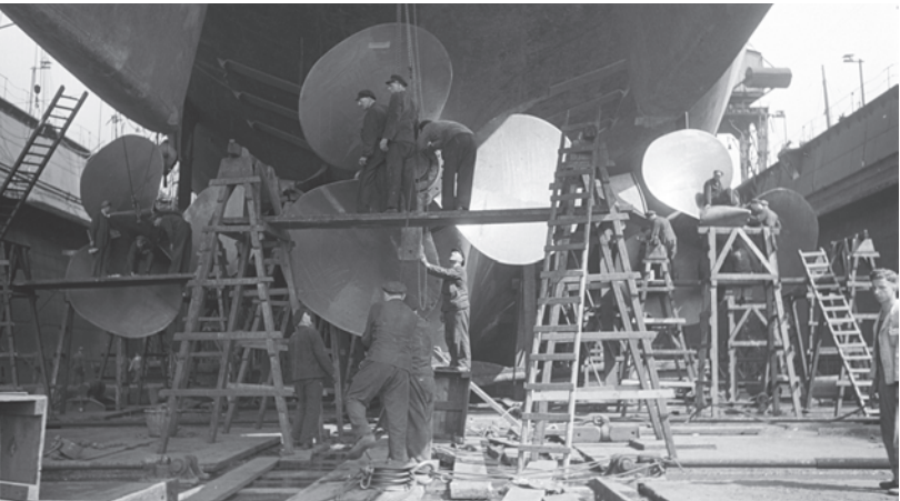
Blohm & Voss shipyard, Hamburg, late June – early July 1940. During her stay in the dry dock, Bismarck had her propellers fitted. As is visible in this photo, the starboard propeller is right-handed (it rotates clockwise for forward motion of the ship), whereas the middle and port propellers are left-handed (they rotate anticlockwise for forward motion of the ship). The lower fragments of both rudder blades are visible above. (Bundesarchiv, Bild 193-30-5-31A)
