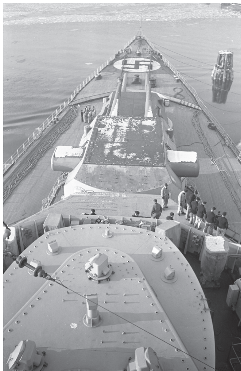
Blohm & Voss shipyard, Hamburg, January 1941. This photo was taken from searchlight deck level looking forward. An antenna insulator is visible in the foreground to the left. Below it, the armoured roof of the conning tower can be seen, with its periscopes and target givers. Further down, the open navigation bridge can be seen, with all kinds of equipment fitted. The roofs of both main artillery turrets are painted dark grey. Turret 'Anton' has its rangefinder already removed. On the forecastle, a large painted swastika is visible – an air recognition sign for friendly aircraft. This was a harsh winter – note the floating ice in the upper part of the photo. (Bundesarchiv, Bild 193-07-1-13)
