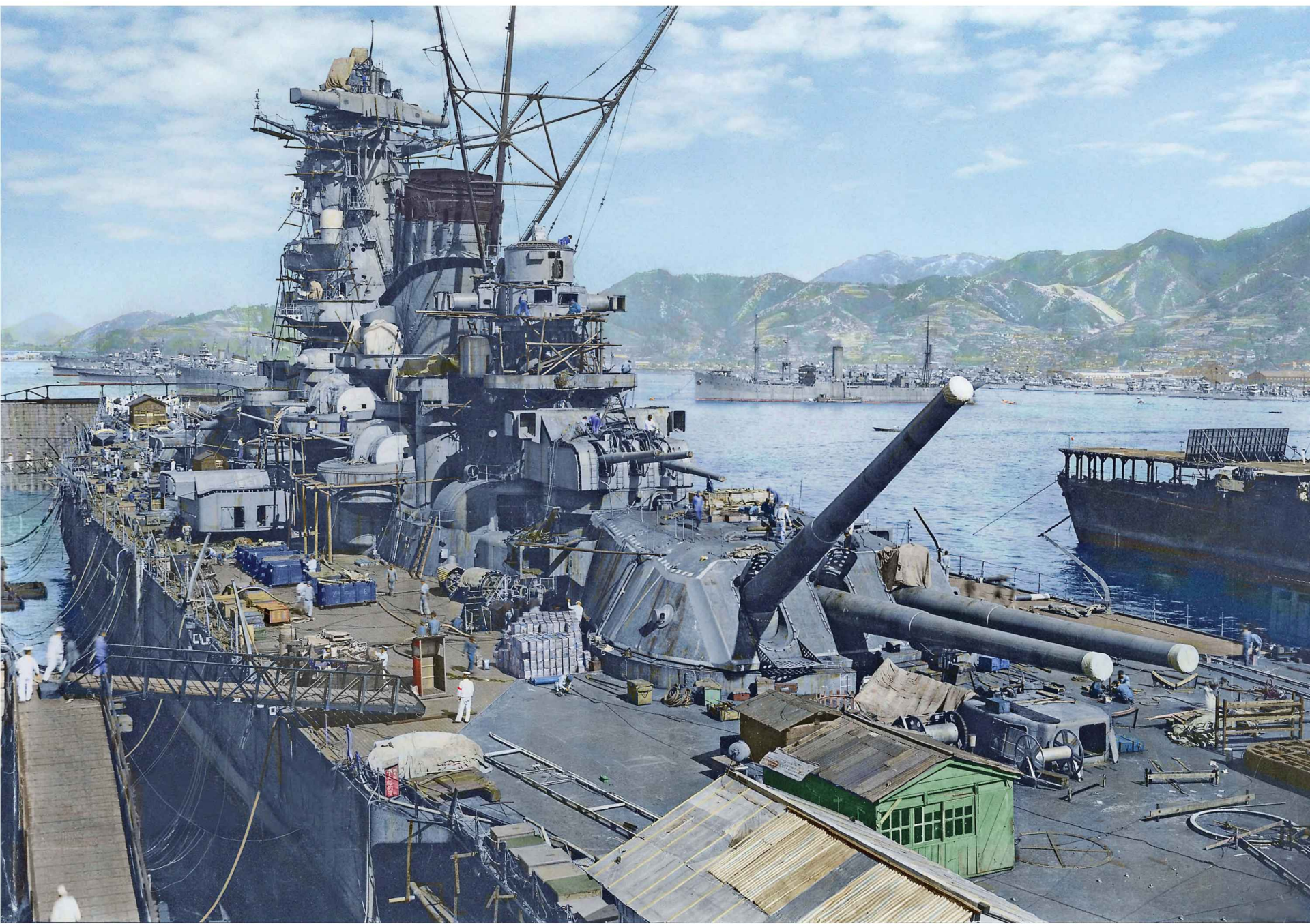
Kure – 20 September 1941 – Yamato is shown during her final phase of fitting out. The steel mesh supports for the canvas blast bags can be seen above and below the nearest gun barrel, and splinter armoured protection below the gun
