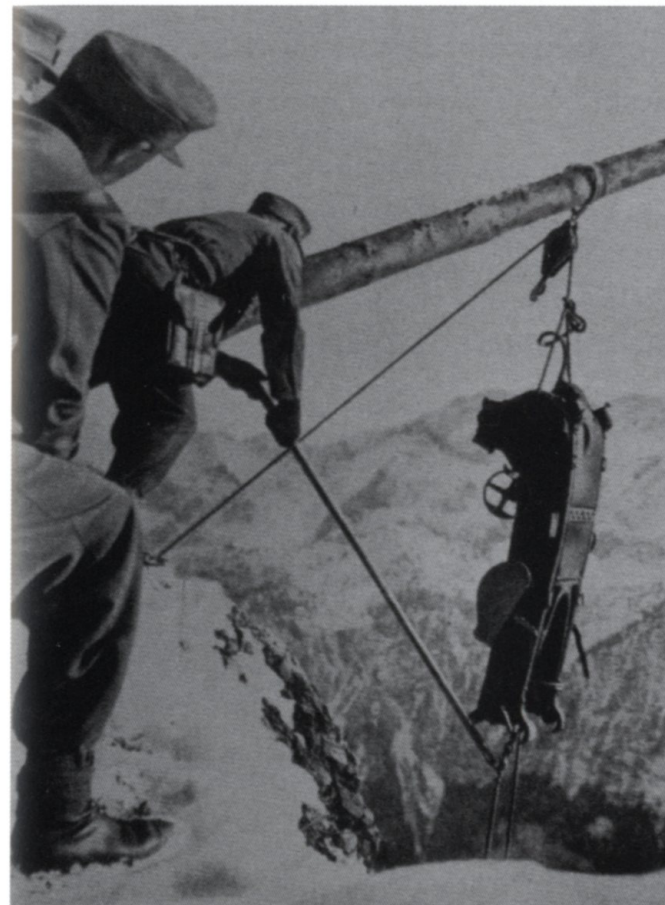
Below: A tree trunk has been called into use with a block and tackle to haul a K15 gun to its firing position.
