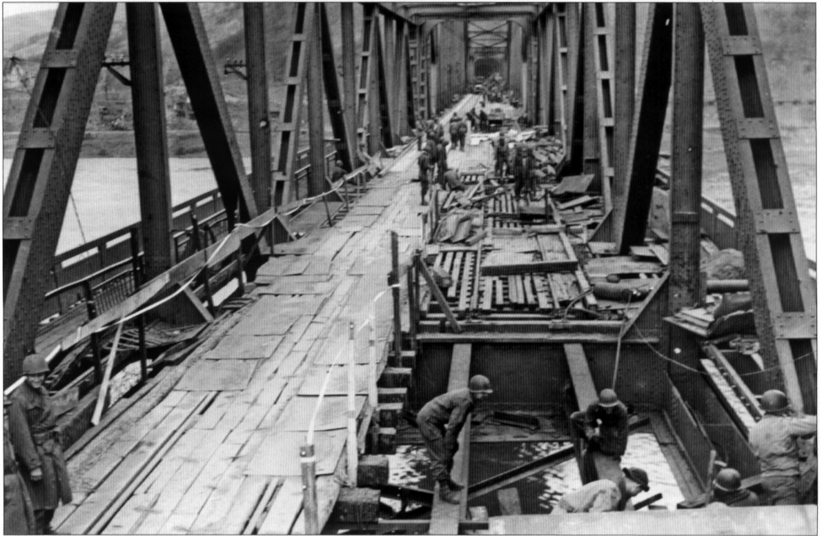
US Army engineers attempt to repair the damage caused to the bridge by the detonation of one of the charges under the eastern pier. This area was further damaged on the night of March 7-8 when a US tank destroyer slipped into the gap while crossing the bridge. (NARA)
