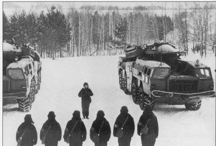
On the final production variant of the 9P117, there is a row of vents on the compartment side over the first wheel, identical to the panel and early and intermediate production 9P117Ms.
