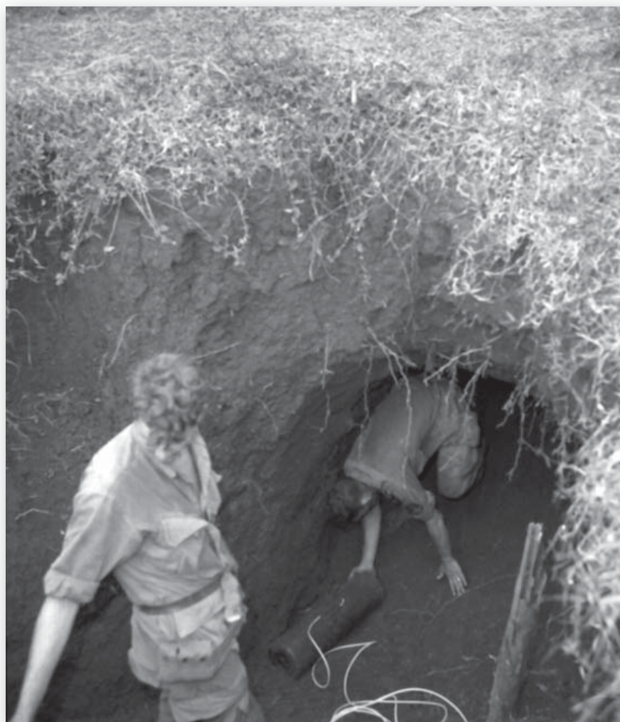
A 40lb cratering charge is dragged into a tunnel by 173rd Airborne Brigade tunnel rats. The amount of detcord indicates that it will be emplaced a good distance inside. (Tom Laemlein/Armor Plate Press)
