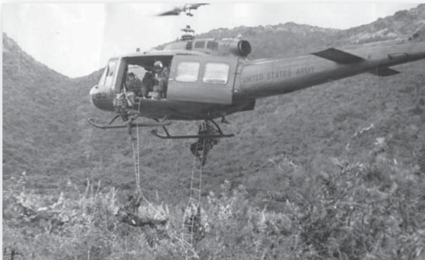
A recon team conducts training using an early type of ladder to board a hovering UH-1H helicopter. This type of narrow ladder proved to be more difficult to climb and descend than the wider ladder introduced later. (Warren Calkin via Steve Sherman)
