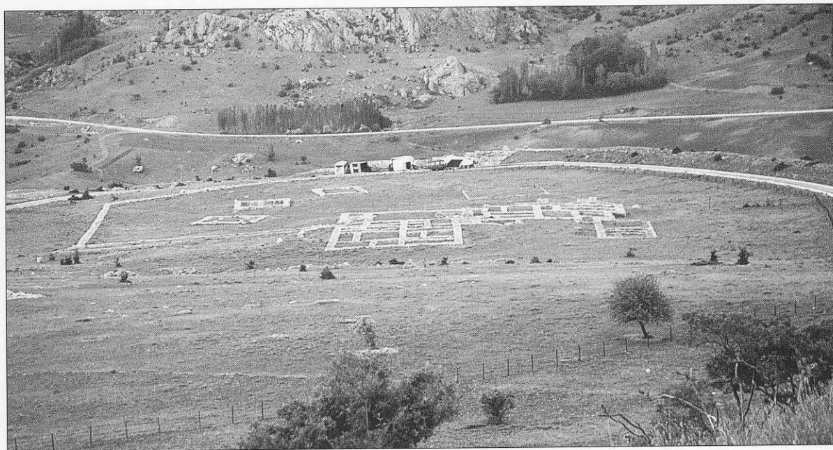
The 'Temple 5' complex in Hattusa, which lies close to the King's Gate. It includes what have tentatively been identified as a palace-annex and three small chapels. The king may have spent his final hours in this precinct, communing with his gods and his ancestors, before setting forth on a military campaign.
