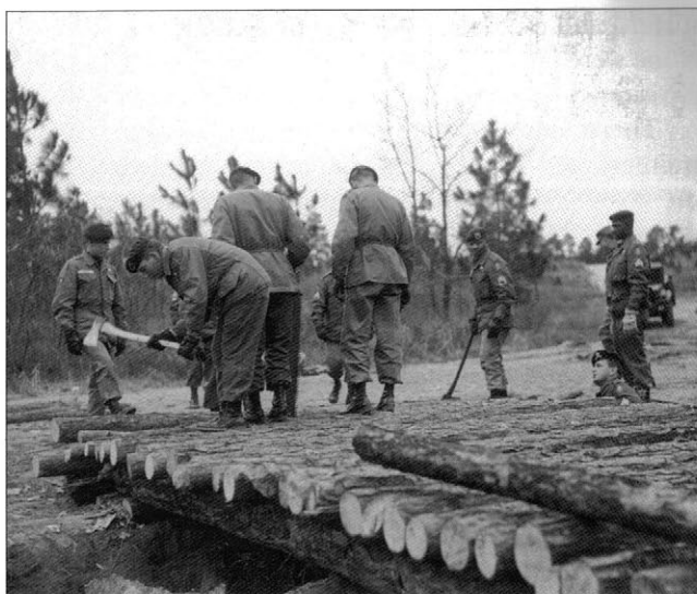
SF training focused on the practical as well as the technical. Here a group of engineers attempt to construct a bridge with only hand tools. They would later destroy it as part of their demolitions training.
