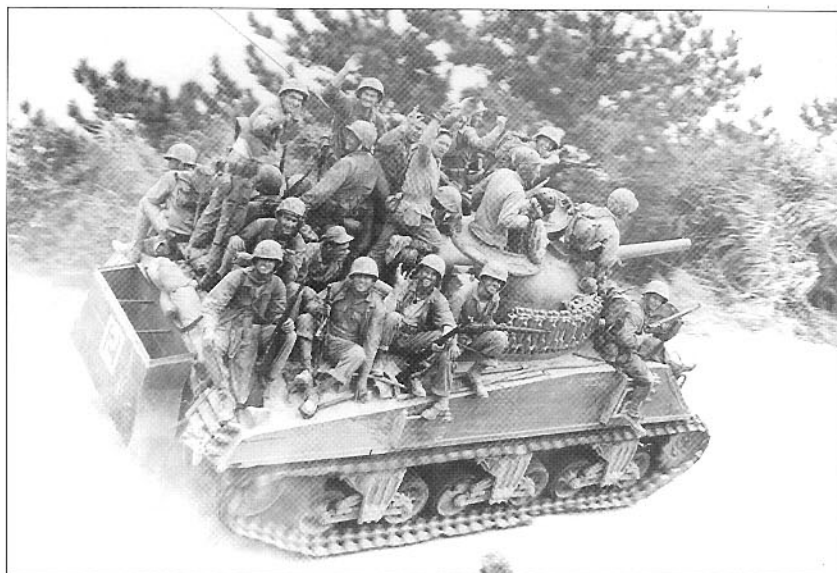
Marine riflemen advance jubilantly to the east and north after landing on Okinawa riding on an M4A3 tank of the 6th Tank Battalion. The lower exhaust section of the fording stacks remains on the tank. Note the excellent vision ring now part of the tank commander's hatch. (USMC photo)
