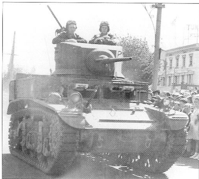
An M3A1 of 1st Tank Battalion parades in Australia, April 1943, where the division refitted after Guadalcanal. The sponson machine guns had disappeared with this model, but the tight fit for a crew of four remains evident. (USMC photo)
