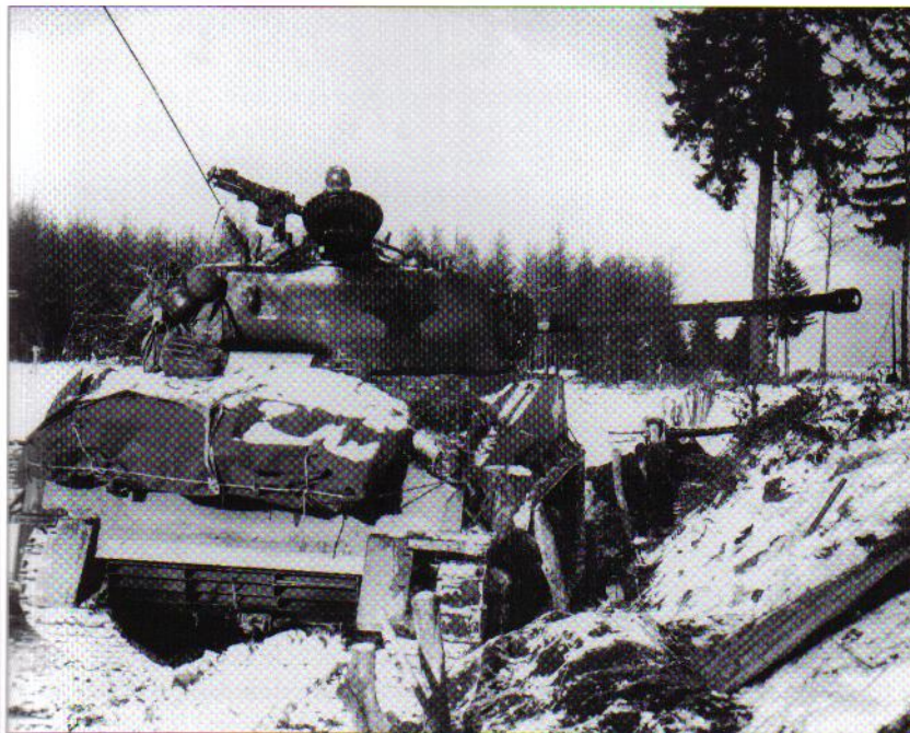
The 4th Armored Division was the first unit in the ETO to deploy the new M4A3E8 tank in combat, with the 37th Tank Battalion receiving a small number in December to replace earlier losses. This version had a new suspension with better traction in snow and mud, and one is seen here in a defensive position along highway H-4 outside Bastogne on January 8, 1945. (NARA)
