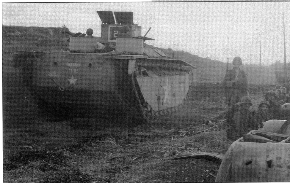
LVT(A)-1 am tanks of the Army's Company A, 708th Amphibious Tank Battalion move past a group of Marines of the 4th Division during the attacks beyond Hill 500 on 22 June 1944. Notice that by this stage of the war, the armored collars around the rear scarf ring machine gun positions have been heightened to provide the gunners with better protection. (USMC)
