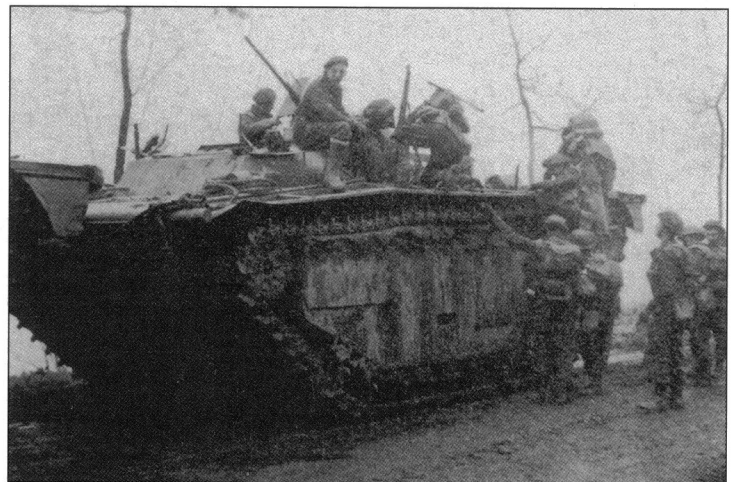
As with the US forces in the Pacific, the British soon learned to add armor shields around the amtrac machine guns. Here, a Canadian infantry unit loads aboard a Buffalo II (LVT(A)-2) during the operations in the Scheldt estuary. The first Buffalo operations against Terneuzen were conducted by the Highland Light Infantry of Canada and the North Nova Scotia Highlanders. (USNA)
