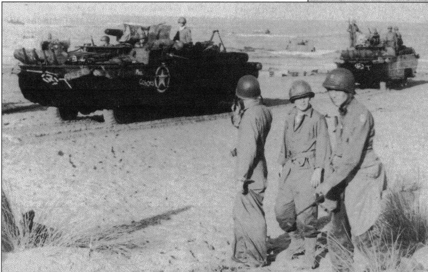
A DUKW supporting the 143rd Regimental Combat Team lands in Italy on 9 September 1943 during the Salerno operation. This unit is bringing a 105mm howitzer battery ashore. The howitzers could then be unloaded using skids carried inside the DUKW. (MHI)
