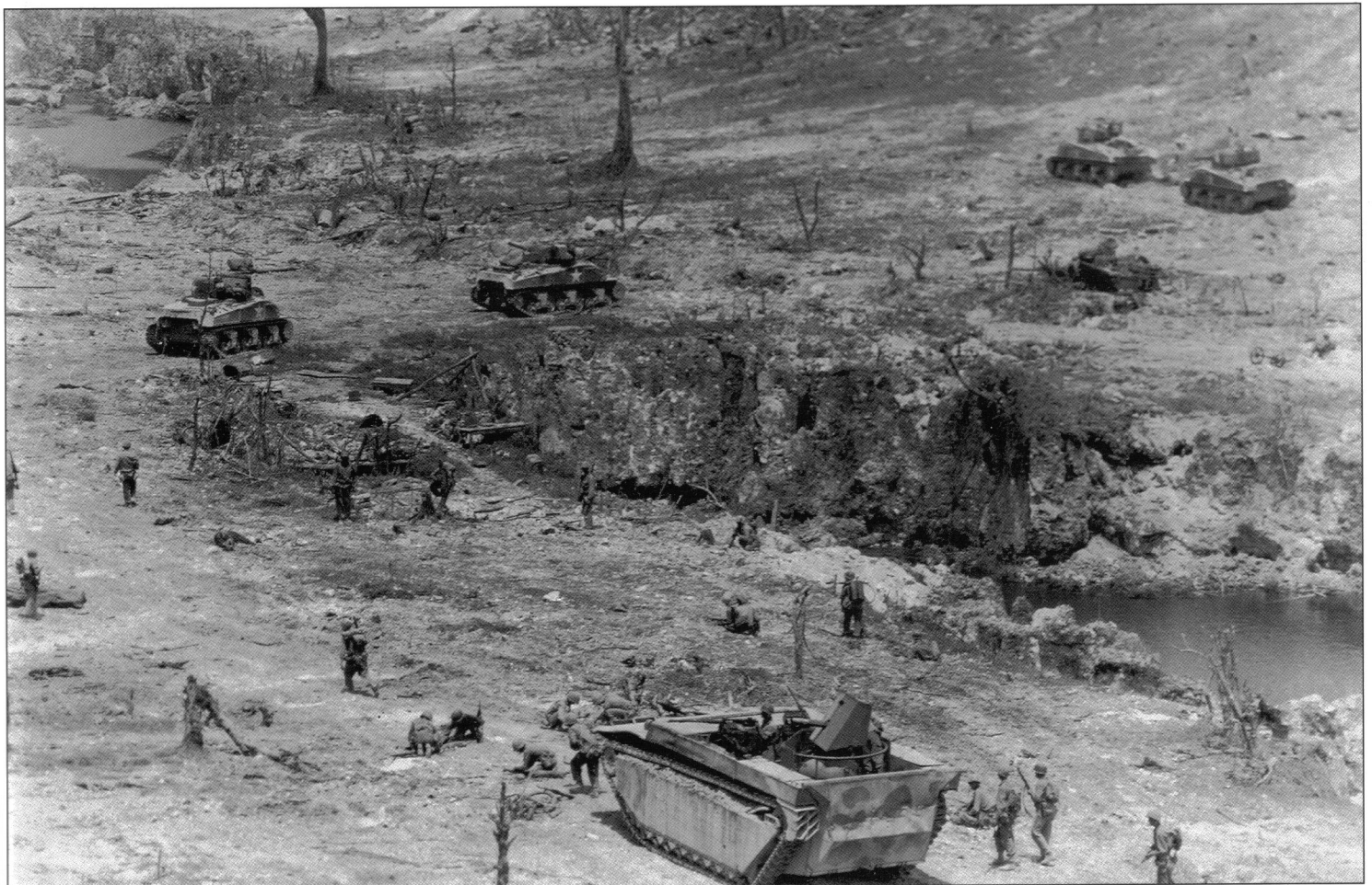
An armored assault on Peleliu halts while Marines remove a massive 200 pound land mine found in the path of one of the LVT-4 flame-thrower amtracs. In the background are M4A2 tanks from the Marine 1st Tank Battalion. (USMC)
