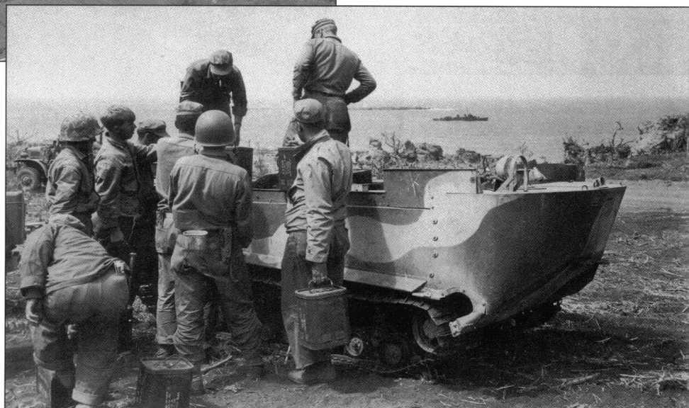
Marines do maintenance on a M29C Weasel on Iwo Jima. These small amphibious utility vehicles were more common in the European theater than in the Pacific. (USMC)
