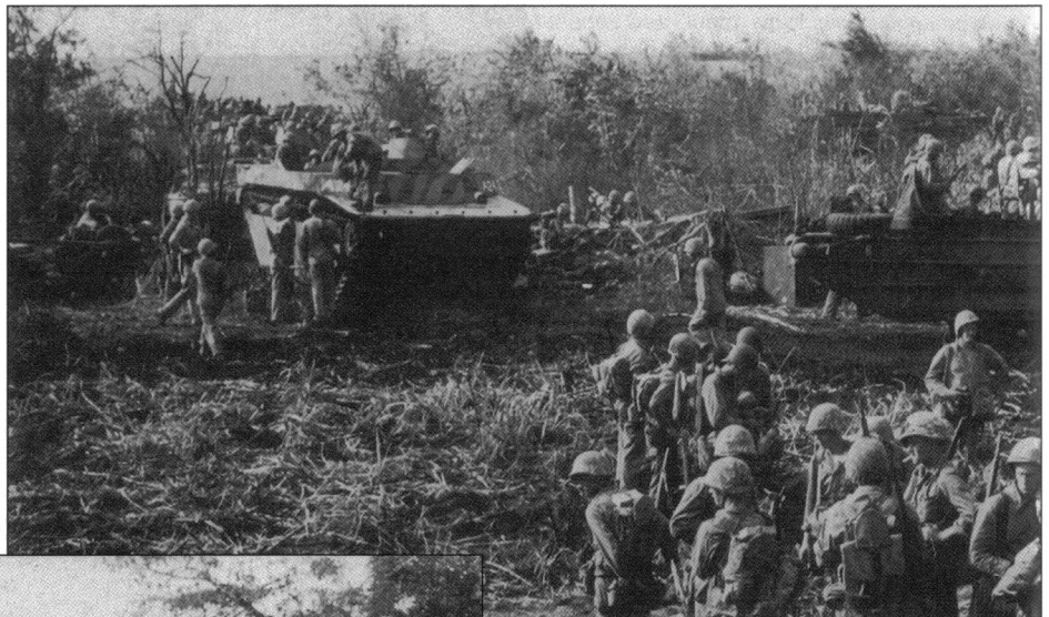
A Marine LVT(A)-4 of the 2nd Armored Amphibian Battalion on Tinian in August 1944. The two turret machine guns have had improvised armored shields added. In addition, the vehicle has pattern painted camouflage. (USMC)
