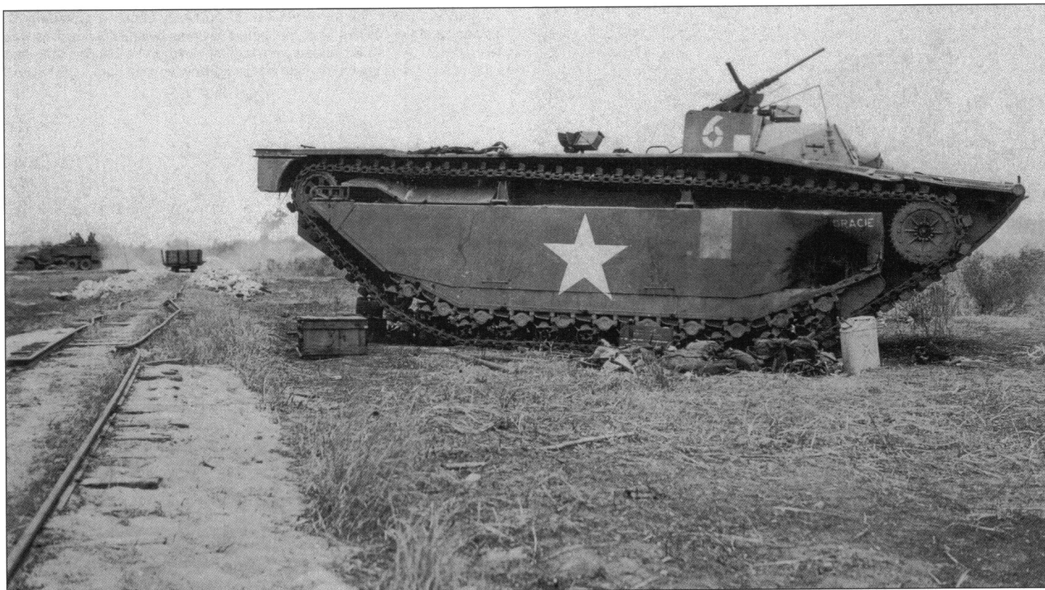
An Army uparmored LVT-2 on Saipan, probably Yellow Beach 1. The amtrac has been hit by an artillery round on the front of the pontoon, creating a large hole under the vehicle name "Gracie". (USMC)
