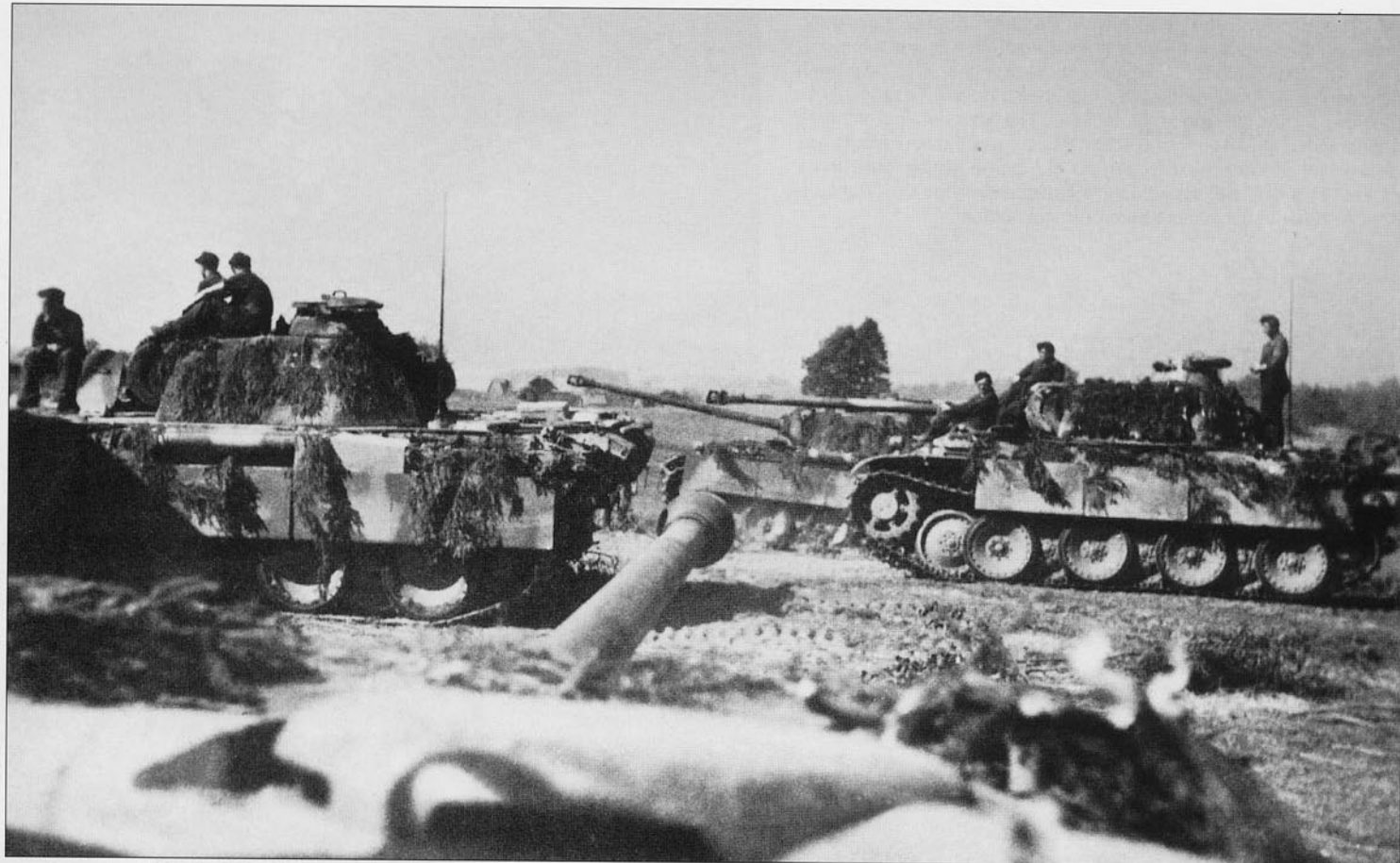
A group of 'Panther' Ausf.G as seen from the turret of another 'Panther'. All of the vehicles have been camouflaged with spruce boughs in addition to their standard camouflage paint schemes. Note the open driver's hatch on the 'Panther' on the left shows the camouflage pattern has been painted on the top of the hull. The dark spot on the roof of the turret in the foreground is the shadow of the vehicle commander.
