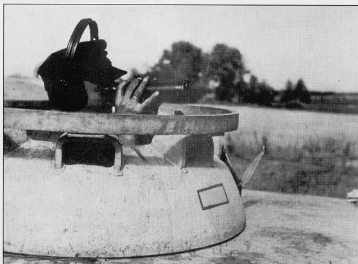
The details of the cupola can be seen clearly in this photo of a 'Panther' commander as he views the terrain ahead through his field glasses. The significance of the rectangle painted below the episcopes is unknown.
