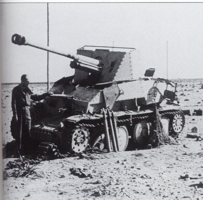
Two photos of a Marder III disabled by a mine blast that has blown off one of the roadwheels and broken the track. These vehicles were armed with captured Russian 76.2mm M1936 field gun, designated FK296 by the Germans, the same gun that was installed on the 'Diana'. It was redesigned and chambered to take the German PaK 40 ammunition. Markings are limited to a black and white national cross painted on the sides and on the smoke hoods on the rear of the vehicle.
