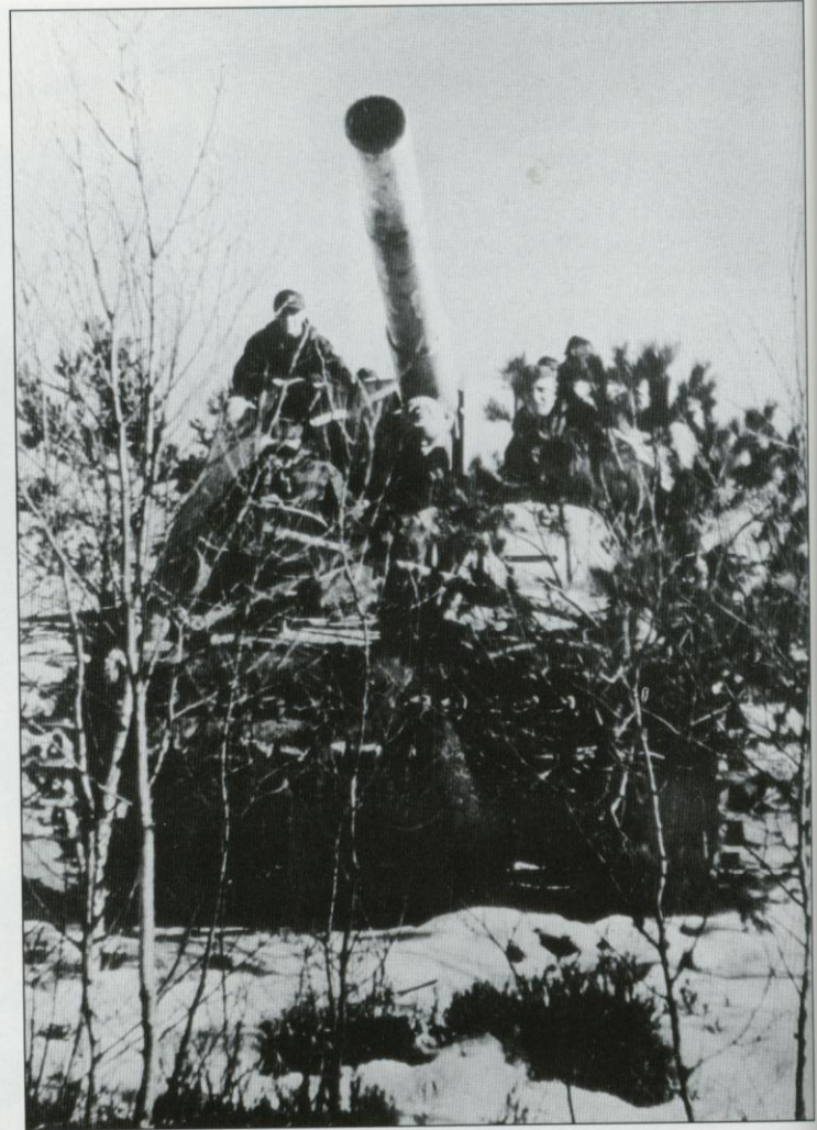
A Hummel has taken up a position in some trees and is ready to go into action. The armament of this self-propelled howitzer was the s.FH 18/1 L/30, which could fire shells at a range of over 10 km (6.2 miles). The main problem with the Hummel was the small capacity of the combat compartment, which could carry only 18 howitzer shells. It was for this reason that the Germans produced many ammunition carriers ( Munitions Fahrzeuge ) based on the same chassis. From the beginning of the Hummel production up to 12th May 1943, 100 self-propelled howitzers and 157 ammunition carriers were produced.
