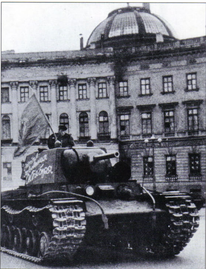
A view of the opposite side of the KV-1 Model 1941 with the uparmored welded turret passing the Winter Palace in the background. The turret slogan is the same as in the other view of this tank. The principal feature of this turret will be noted by careful inspection of the area in front of the turret overhang immediately left of the first letter of the third line of the slogan. Notice also that this vehicles are beginning to sport a layer of appliqué armor on the hull front and hull sides.
