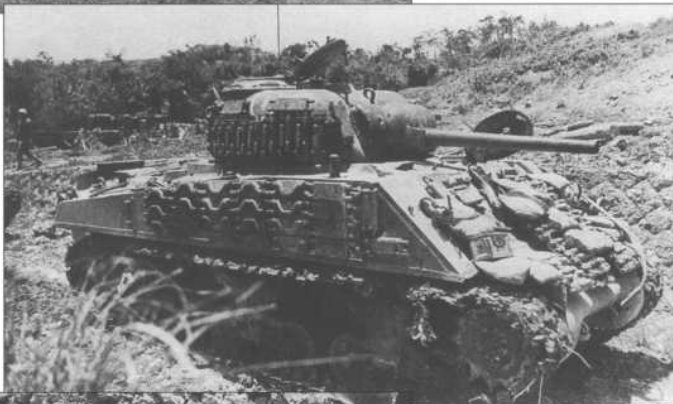
A Marine M4A2 (W) medium tank of the 1st Marine Tank Battalion on Okinawa. This is one of the late production types with the new commander's all round vision cupola. This unit painted its tactical insignia on the upper edge of the turret due to the use of extensive track blocks, in this case a circled number 1.
