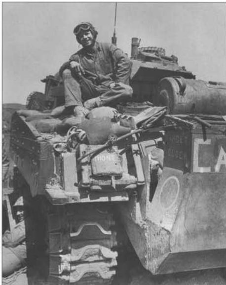
This close-up view of the rear end of "Calcutta", a M4A2 (W) of Co. C, 4th Tank Battalion, shows many small markings details. The Target Clock painted on the wading trunk was intended for Marines using the infantry phone attached nearby. This was to remind them to call out targets using the clock method to identify directions. The fuel container on the deck has apparently been rigged for carrying water, with a spigot mounted near the tank phone. Notice also that the tank name is repeated on the rear of the wading trunk.
