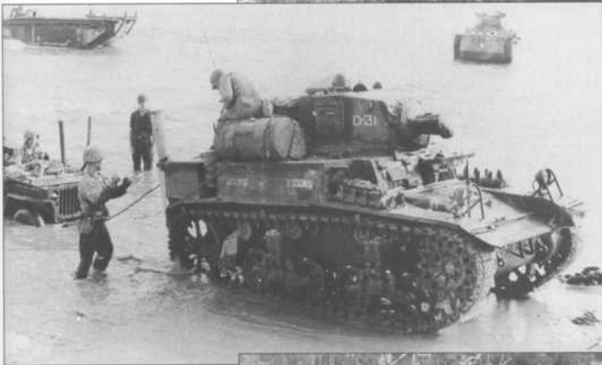
"Ding Dong", a M3A1 Satan flamethrower tank of the 2nd Tank Battalion is landed on Saipan on 25 July 1944. Notice that an improvised tube has been added instead of a standard deep wading stack.
