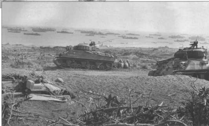
With the experiences of previous campaigns, Marine tank deployed on two Jima in February 1945 were well prepared to deal with Japanese infantry anti-tank tactics. This M4A2 (W) of the Marine 5th Tank Battalion has planking on the side to prevent the attachment of magnetic mines, and penny nails welded to the turret hatches to prevent the attachment of satchel charges intended to blow open the hatches. This tank became bogged down near the landing beaches in the soft volcanic soil.
