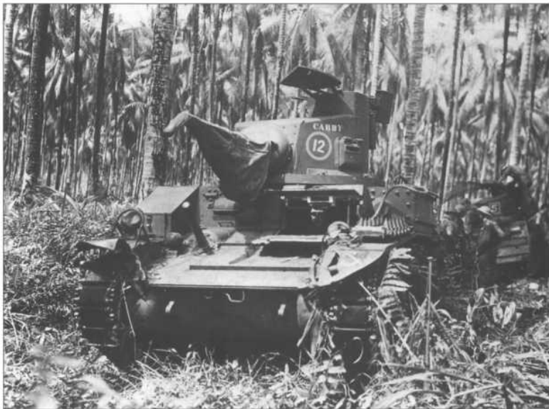
A rear view of a disabled Australian M3 Stuart light tank disabled when it became stuck on a downed coconut tree during the fighting on Cape Endaiadere in late December 1942 while attacking a series of Japanese bunkers. Several interesting details can be seen on the photo including the use of track grousers to improve traction in the jungle, the open lids of special stowage bins added by the Australians to these tanks, and the 1st Australian Armoured Division insignia on the right corner of the rear engine deck.
