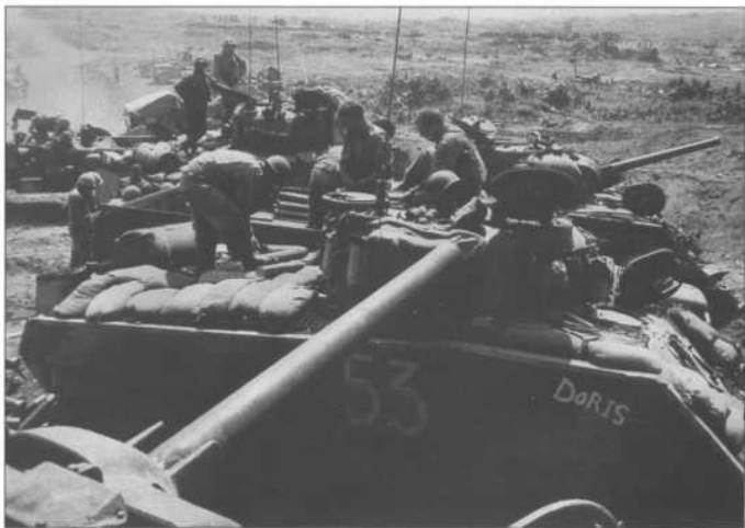
A M32 armored recovery vehicle in the foothills of Mount Suribachi. The soft volcanic soil of the island meant that these vehicles were often put to good use. The American flag raised on Mount Suribachi can barely be seen in this view.
