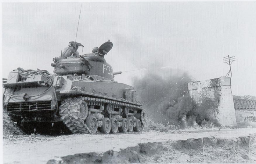
One curious improvisation on some Marine M46s in the final months of the fighting were these improvised casing catchers mounted on the left side of the turret near the loader's hatch. These were intended to catch the spent ammunition casings. So much ammunition was expended during artillery fire missions, that the basket was more convenient than having to police up the area for spent casings after each fire mission.
