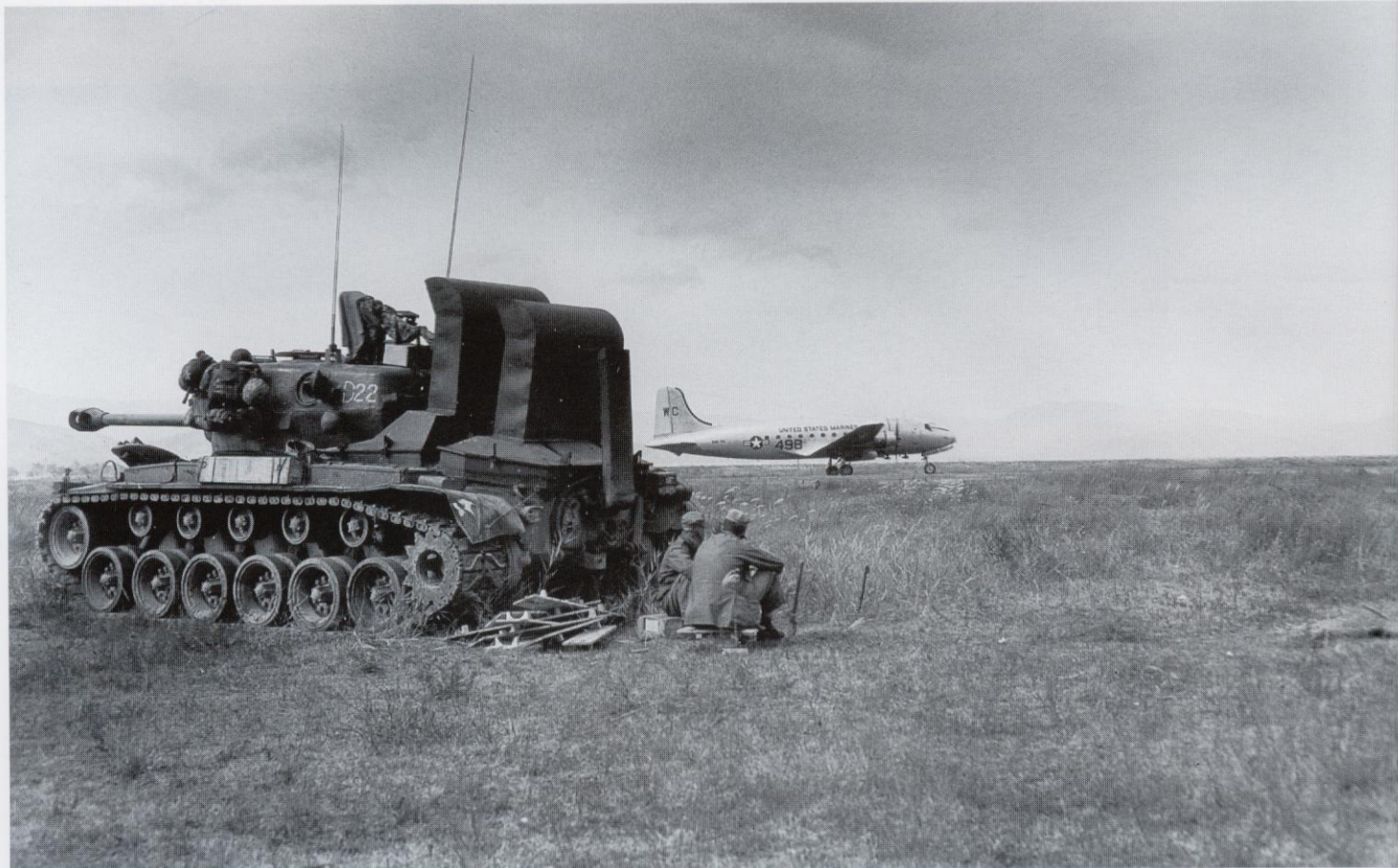
On 27 October, another amphibious landing was conducted at Wonson, on the eastern coast of Korea by the 1st Marine Div. By this time, the NKPA was in total disarray, and the landing was unopposed. The M26 tanks of D Co., Marine 1st Tank Bn. were fitted with the full deep wading trunks for the operation to allow the tanks to be landed in the shallow harbor from LSUs. Here, one of the tanks sits near the airbase with its wading trunks still attached.
