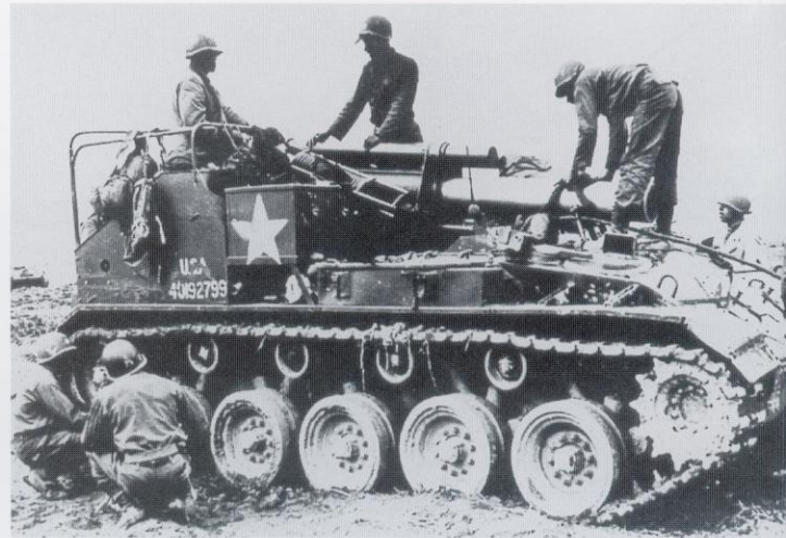
Another derivative of the M24 was the M41 155mm howitzer mortar carriage. This vehicle was a combination of the M24 light tank chassis with the M1 155mm howitzer. This particular vehicle served with the 999 Field Artillery of the 24th Infantry Div.
