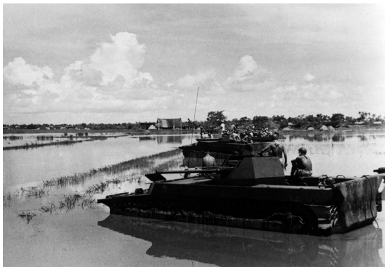
Mounting 40mm Bofors guns, Alligators of 6e GEA/1er RCC form a 'bouclage' (cordon) near Nam Dinh, 1953. A number of LVT4s were fitted at Haiphong naval arsenal with an open-topped turret mounting a Bofors for the fire-support role. These vehicles were only employed by the amphibious units of 1er RCC – note the regimental insignia well forward on the hull sides. They proved effective in the Tonkin deltas, but the increased weight and height affected their seaworthiness, so they were rarely used in amphibious coastal assaults. With no threat of air attack, the equipment of the Artillerie Antiaérienne Légère units was distributed for other purposes; 40mm Bofors guns were deployed on armoured trucks, armoured trains and LVTs. (Author's collection)
