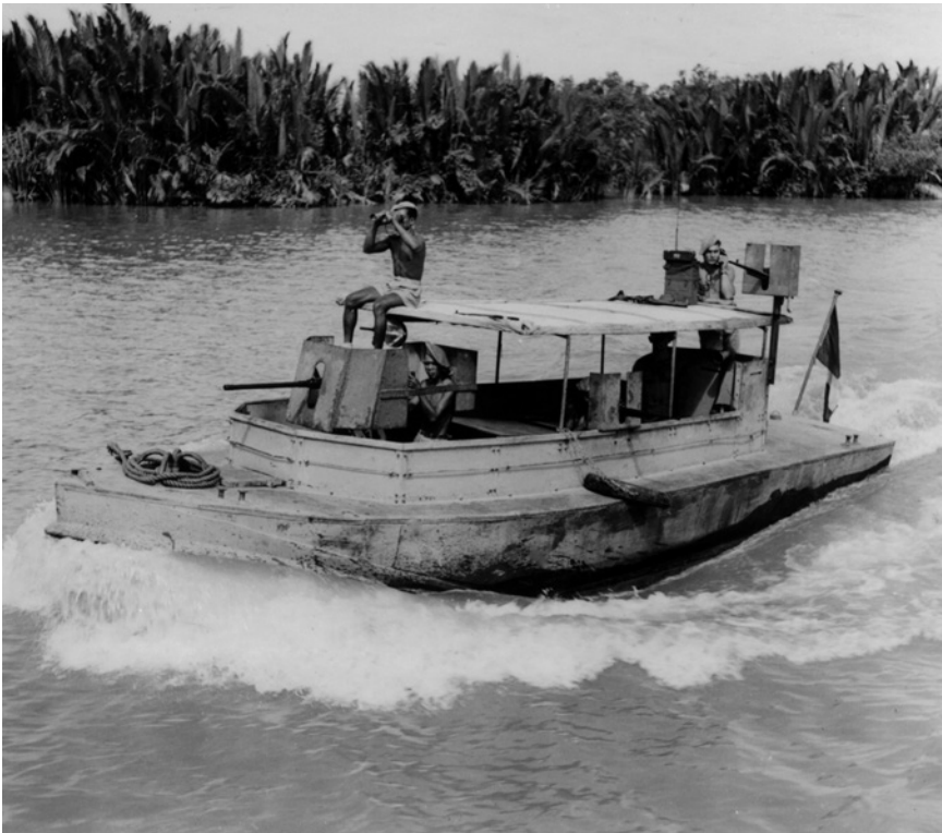
Vedette FOM (France Outre Mer) manned by dragoons from the 4e RDP, escorting junks carrying rubber from the Michelin plantations along the Saigon River. These armoured motor boats, able to navigate narrow creeks in pursuit of enemy sampans, came in two sizes, 8m (as here) and 11m long; the former was usually armed with one .50cal Browning and two or three Reibel 7.5mm machine guns, together with rifle-grenade launchers. Five or six crewmen were drawn from armour units, such as the 4e RDP, RICM, 5e RSM and 1er REC. At the end of the war, 89 Vedettes were in service in all parts of Indochina. (Author's collection)
