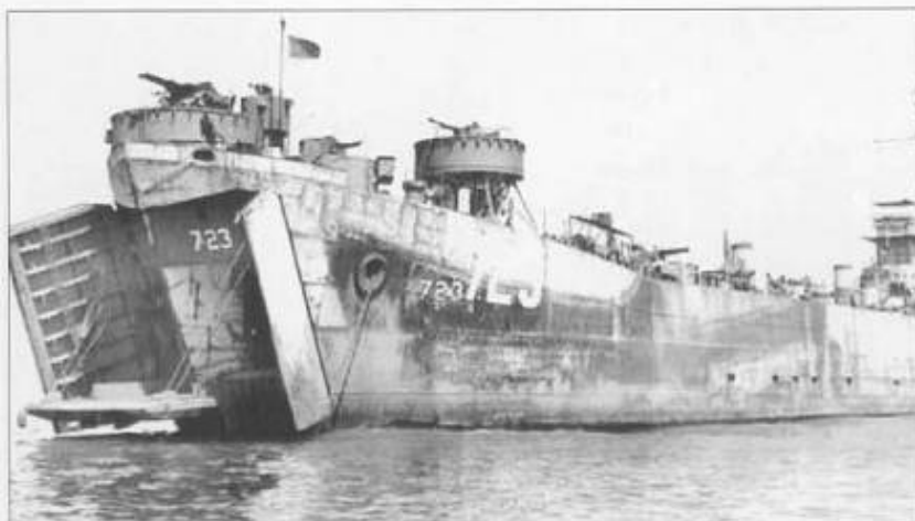
An unballasted LST-723 cruises with its lowered ramp above water. She has seen hard service judging from her deteriorating Tropical Measure 31/17L dappled edge scheme. This photograph was probably taken after it had participated in back-to-back operations at Iwo Jima and Okinawa. In 1944 6ft hull numbers were directed and time did not even allow the former 2ft numbers to be painted over.
