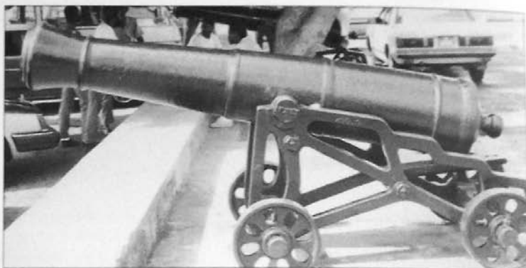
Naval 18-pdr iron model 1778 gun. This gun was cast in 1785 at the Indret iron works and marked No. 75. Its companion gun in the background was cast in 1786 and marked No. 130. These guns were preserved at Plymouth, Montserrat, West Indies. (Photo RC)
