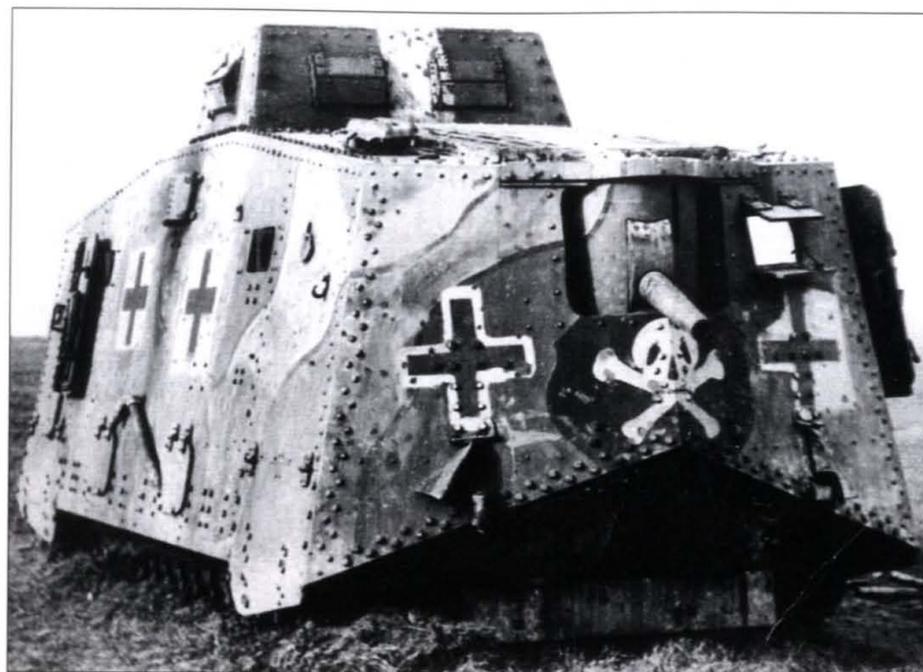
Panzer 503 of Abteilung 3 survived the final fall 1918 battles, but had to be abandoned at Charleroi when BAKP 20 evacuated to Wiesbaden in October 1918. The photo provides a good view of the new markings adopted on October 6, 1918, which were supposed to consist of a Balkan cross on a white square. This A7V was one of the early production batch with the trestle gun mount, later rebuilt with the pedestal mount as seen here. (Patton Museum)
