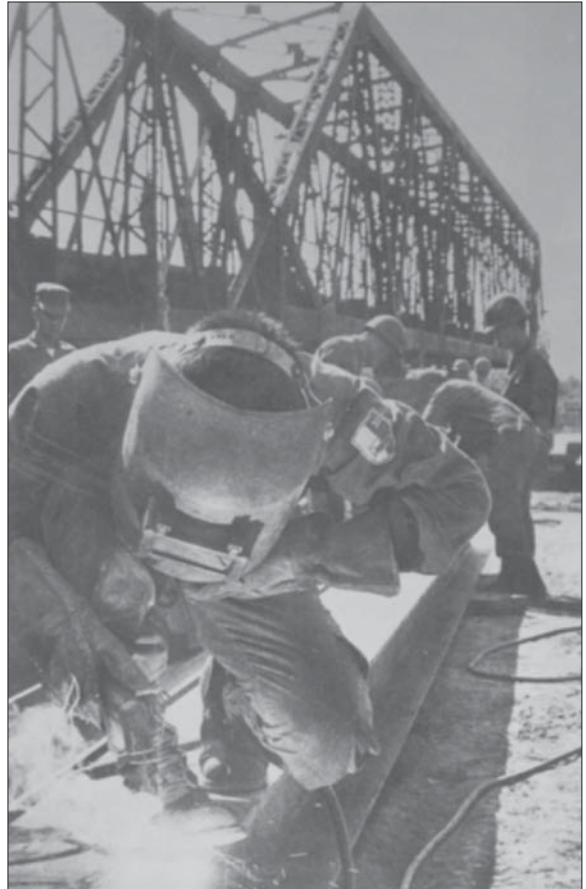
Each ARVN corps possessed a three-battalion engineer group; here a welder of 30 Engineer Bn prepares a beam for the erection of a new bridge as part of the effort to rebuild and reopen the country's highway system. (The French-built railroads had essentially been destroyed by 1962, but lengthy stretches of track also began to be reopened in 1969.) Note the welder's left shoulder patch; engineer battalions all wore halved white-and-red shields, with a black bulldozer in silhouette and a number at top right, basically similar to the design of the artillery battalion patch, which bore a cannon silhouette instead. (Nguyen Ngoc Hanh)
