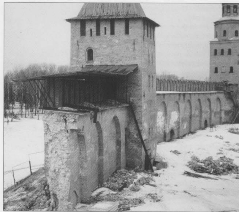
Tower Three of the Kremlin in Novgorod, seen from Tower Four. Tower Three is 15th C, and the broken wall between the towers can be seen to consist of two brick facings filled with a rubble core. (D.Nicolle photograph)
