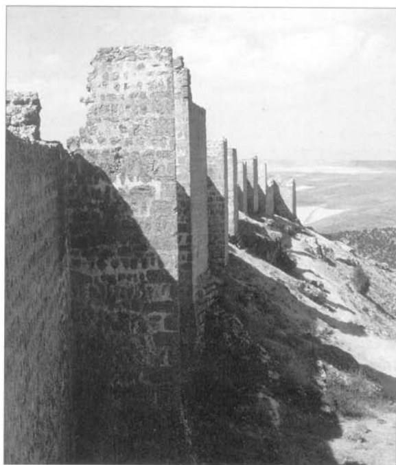
Part of the massive mountaintop castle of Gormaz which, unlike al-Baqar, was a major centre of frontier defence. It is constructed not of concrete but of stone, with 24 closely spaced towers, and encloses the entire summit of a small mountain. It was built in response to the first wave of Christian attacks during the 10th century and guarded one of the main passes through the Sierra de Guadarrama which served as a front line in Andalusian resistance to Christian conquest. (Author's photograph)
