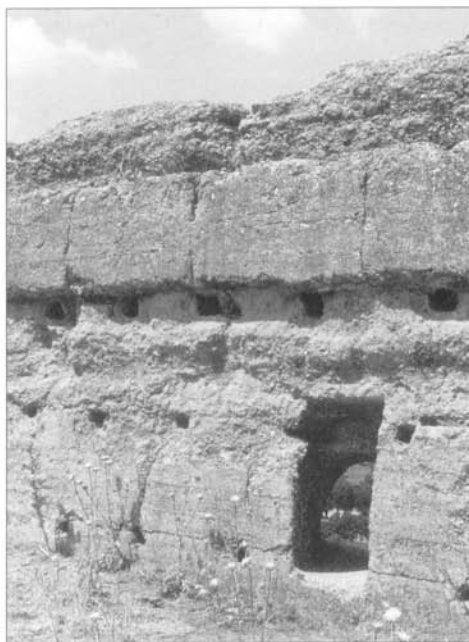
Part of the tabiya or concrete fortifications of the 10th-century castle of al-Baqar north-west of Cordoba. Tabiya was cheap and quick to erect, being laid in wooden shuttering forms which left the horizontal casting lines which can still be seen today. This view of the inside of the wall and a small postern door shows a series of rectangular holes which may have been for an internal wooden walkway. (Author's photograph)
