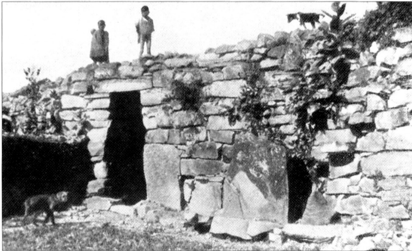
A stone wall at Jotsoma, typical of those which subdivided Naga villages to protect individual clans from one another. Such defences could be several metres thick.
