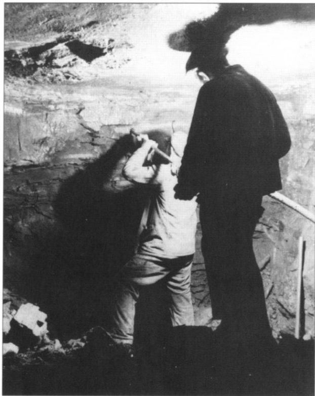
Some of the defences of the West Wall – for example the tunnel systems – were bored into solid rock. This was dirty and dangerous work and those who undertook it were given special pay and allowances. (Bundesarchiv)
