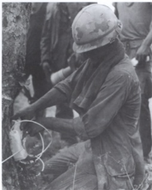
A soldier linking 2½lb M5A1 C4 demolition charges with detonating cord. These will be used to blast down trees to clear a helicopter landing zone, either for a routine resupply or to extract the unit.
