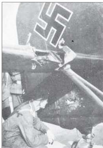
Crewmen inspect flak damage to the tailplane and rear fuselage of an unidentified 'Berta' after a mission over Poland
