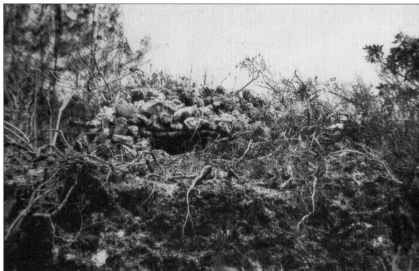
This machine-gun position was constructed of limestone rocks, blended into the surrounding terrain, and well camouflaged with brush. Most of the flamethrower-scorched brush had been pulled away to reveal the position. Such positions were well camouflaged and too small for naval gunfire spotters to detect and had to be reduced by infantrymen.
