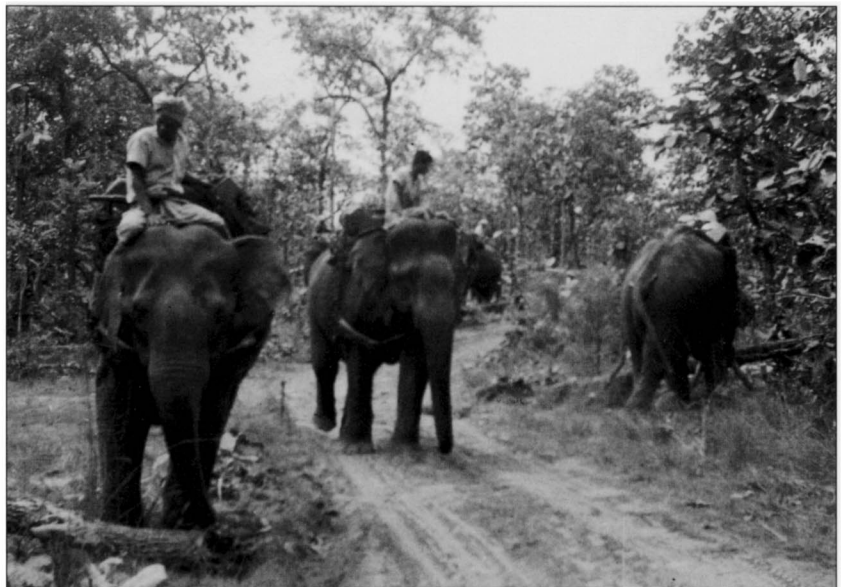
7th Division had to make its own road as it advanced down the Valley. Teams of elephants helped clear the track so that engineers could lay down a temporary road surface. (IWM HU 1079)
