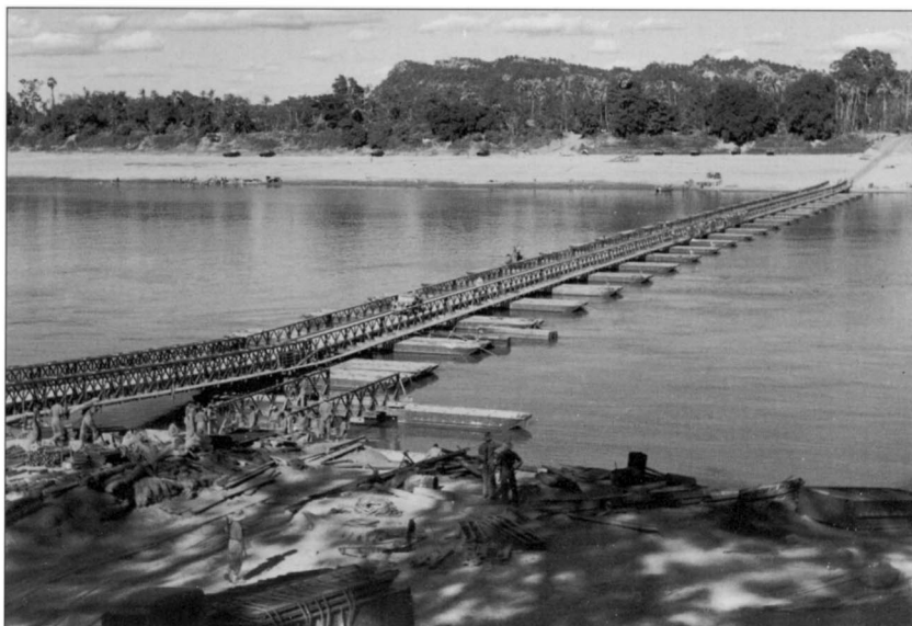
A Bailey bridge across the Chindwin River. At one point this was the longest Bailey bridge in the world. All the sections had to be carried across the mountains to the Chindwin. (IWM SE 2827)
