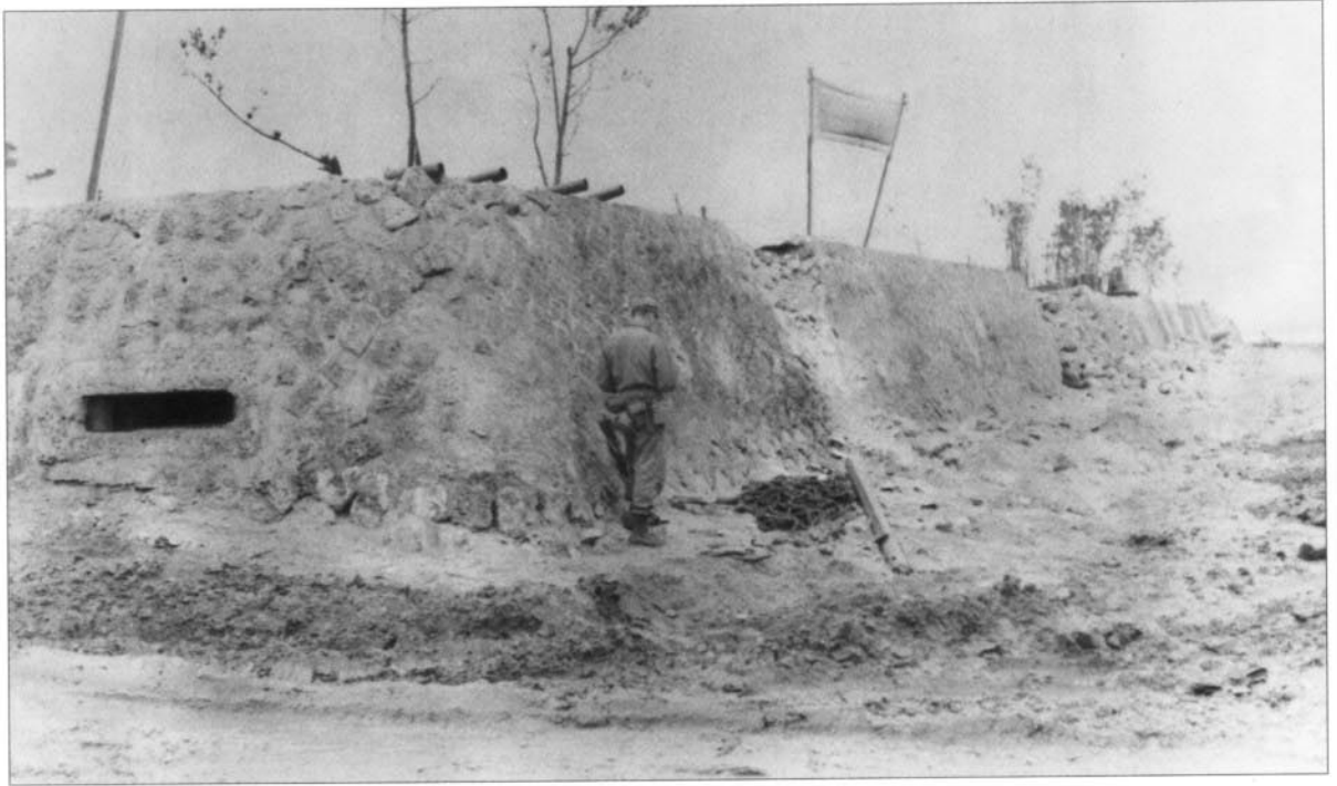
A heavily constructed concrete, limestone, and log bunker line on Mezado Ridge 500–600 yds (455–546 m) southwest of Kunishi and 1,200 yds (1,092 m) south of Itoman, 21 June. While used as bomb shelters, an embrasure was provided for a light machine-gun. Only a direct hit by a large-caliber projectile or a heavy bomb would breach such bunkers. (US Army)
