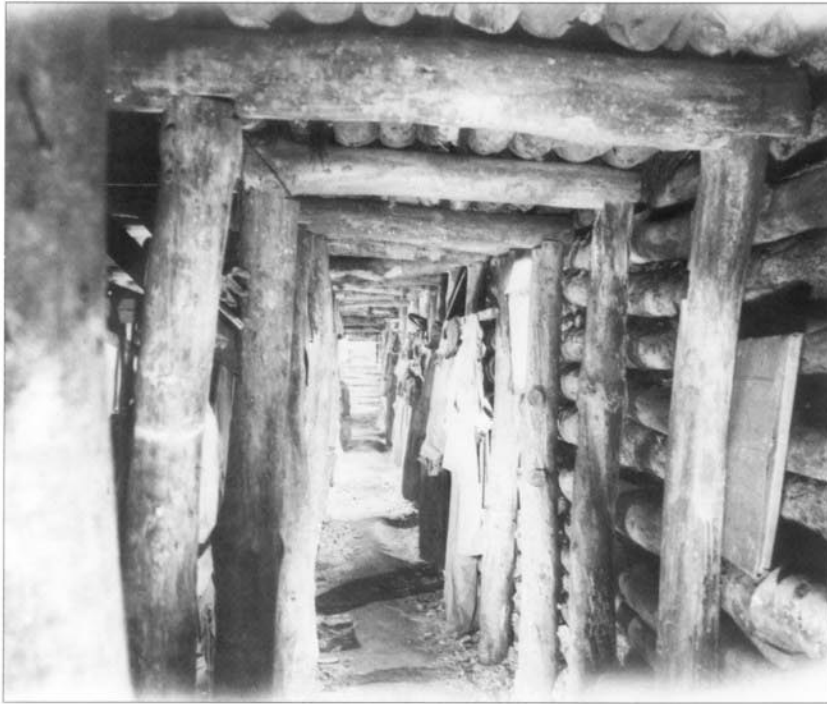
This 100-ft (30-m) long heavily log-reinforced tunnel had five rooms branching off it. The tunnel was found on Ie Shima, but was typical of those on the main island. They served as troop shelters during bombardments, housed command posts, aid stations, ammunition, and supplies. (USMC)
