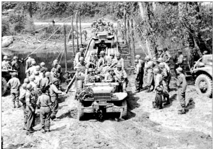
The Vire river had been the eastern boundary of the US advance during Operation Cobra since the main emphasis was a swing westward to trap the Seventh Army. With the encirclement completed attention shifted eastward. This is the first motorized column over the Vire on 3 August after engineers have erected a treadway bridge for the 35th Division.
