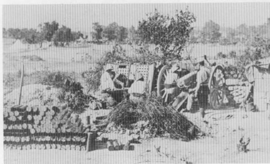
◀ A French '75' in position at the right of the Allied line at Helles. To the left of the gun is the limber, turned upon its side, allowing access to the ammunition through the open top. Two of the crew wear kepis, but the remainder have the distinctively shaped French topee.
