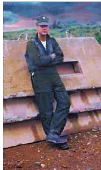
An aviator stands beside prefab contract bunker caps. These were helicoptered into firebases and set over pre-dug, pre-sandbagged bits. (Peter J. Dunne)
