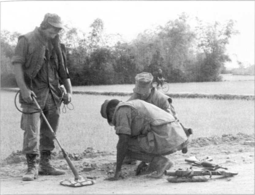
The most hazardous task for the division engineers was the daily sweep for mines planted in the roads each night by VC sappers. The general absence of paved roads made the enemy's task far simpler. (MCRC)
