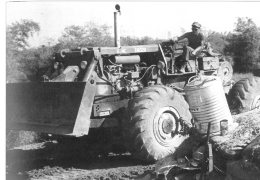
Road and bridge repair and improvement were a constant burden. Here a wheeled dozer from 9th Engineer Battalion works on a bridge approach. Note the water can and weapons close at hand. (MCRC)
