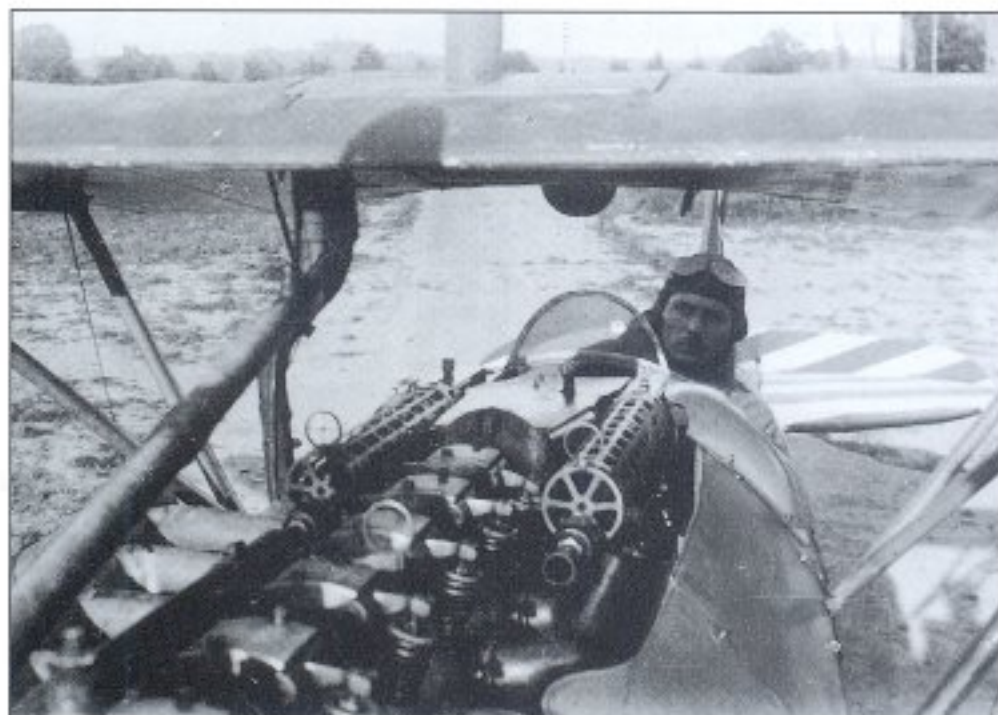
This business end of Hamster's Jasta 37 D III is nicely displayed in this view straight out of a Hollywood film. Note the central radiator and the diagonal black/white stripes on the tailplane, which were the most conspicuous of the unit's markings ( HAC/UTD )
