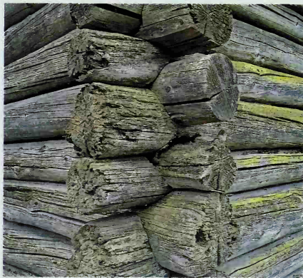
Below This blockhouse construction of horizontal logs with lapped corners is just one of the many different methods of building in wood that were utilized in Viking Age Scandinavia.
