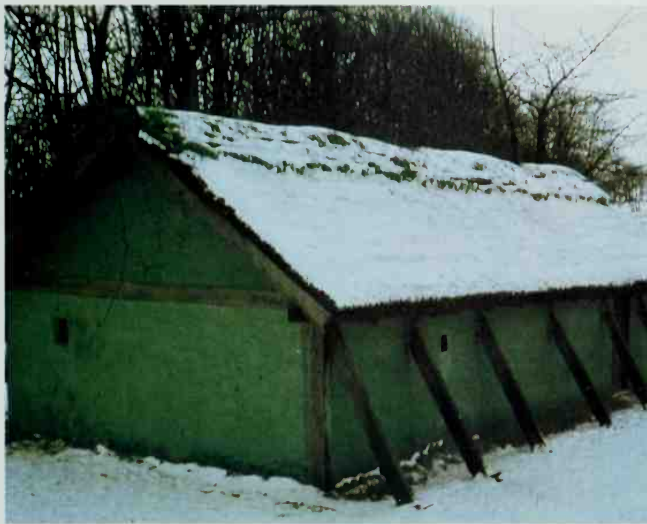
Left This full-size reconstruction of a Viking Age town house from Hedeby stands at Moesgård Museum in Denmark. It measures 12 by 5 meters and has wattle-and-daub walls in a timber framework, with the weight of the thatched roof supported by external buttresses. This Hedeby house, built about 870, had a central living room, between two other rooms, one of which contained a baking-oven.
