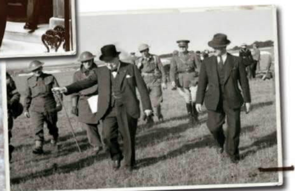
BELOW: On 28 August 1940, Churchill was driving to inspect defences in Kent when a Messerschmitt Me 109 crashed nearby at Church Whitfield outside Dover. Churchill ordered his car to stop and walked over to view the plane with his personal bodyguard Inspector W Thompson (right).
