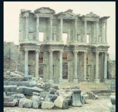
Above: The Celcius Library built at Ephesus, Turkey, by Julius Aquila in 135 CE, after restoration.
