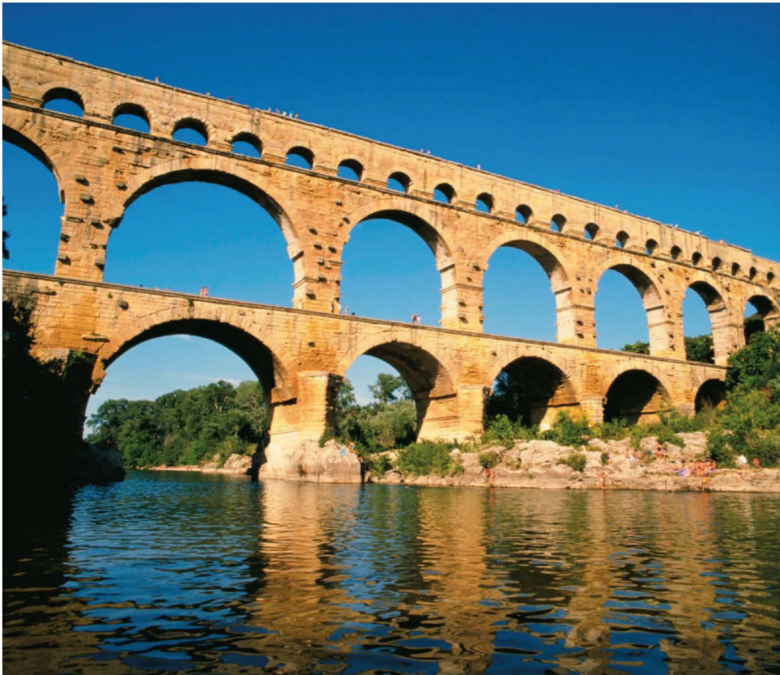
Above: The three-tiered Pont du Gard crossing the River Gard as it takes water from Uzes to Nîmes in France.
